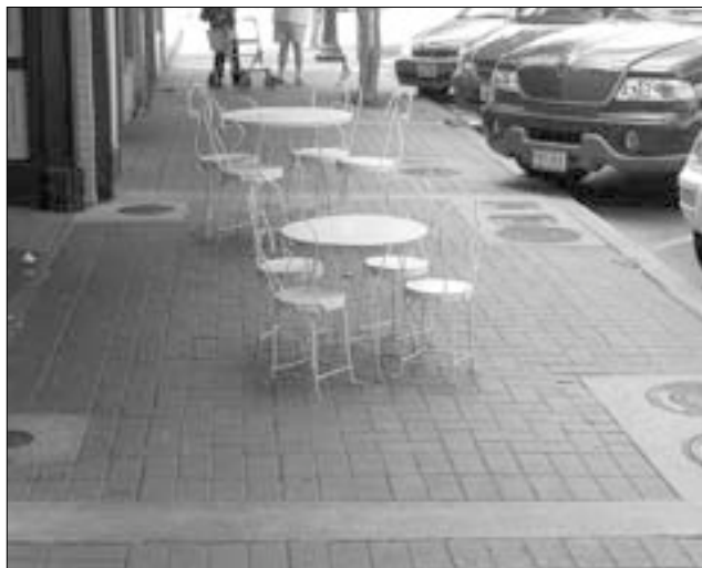
Example of a Level I sidewalk. (Georgetown, TX)
